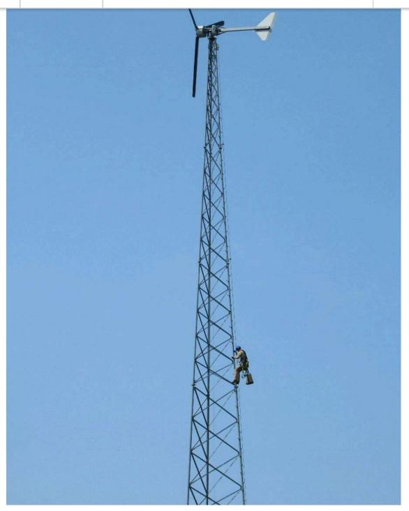
Our wind turbine, which for 10 years supplied most of the power used by the farm, has been out of commission since 2020. Since then we've had a few false starts with companies we contacted to repair it. This week we found a company willing to take on the task. Shown here is one of the workers from Storke LLC repelling down the 120 foot tower after throroughly inspecting the turbine. .We are hopeful that they will be able to get it producing power again before year's end.
